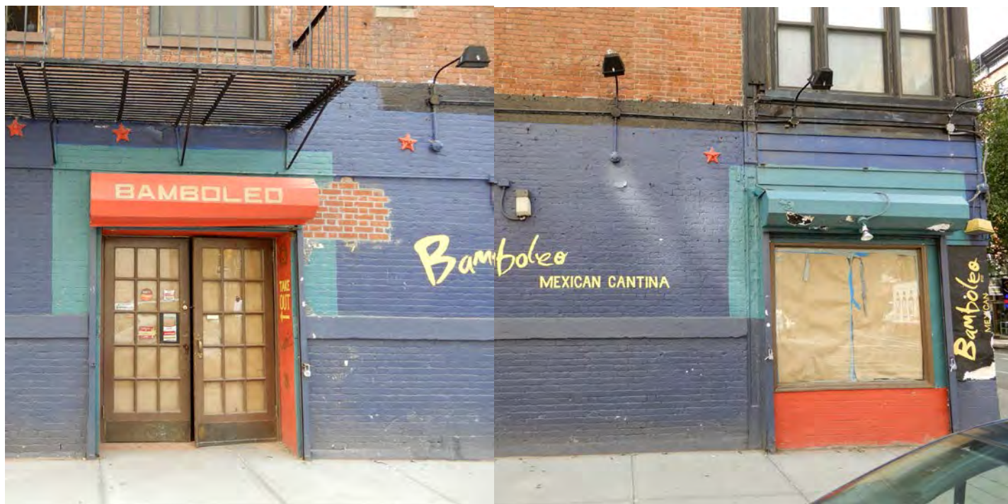
Corner Storefront at North & Double Doors
